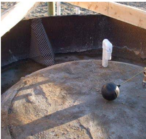
Older tanks can be retro-fitted with ramp inserts.
