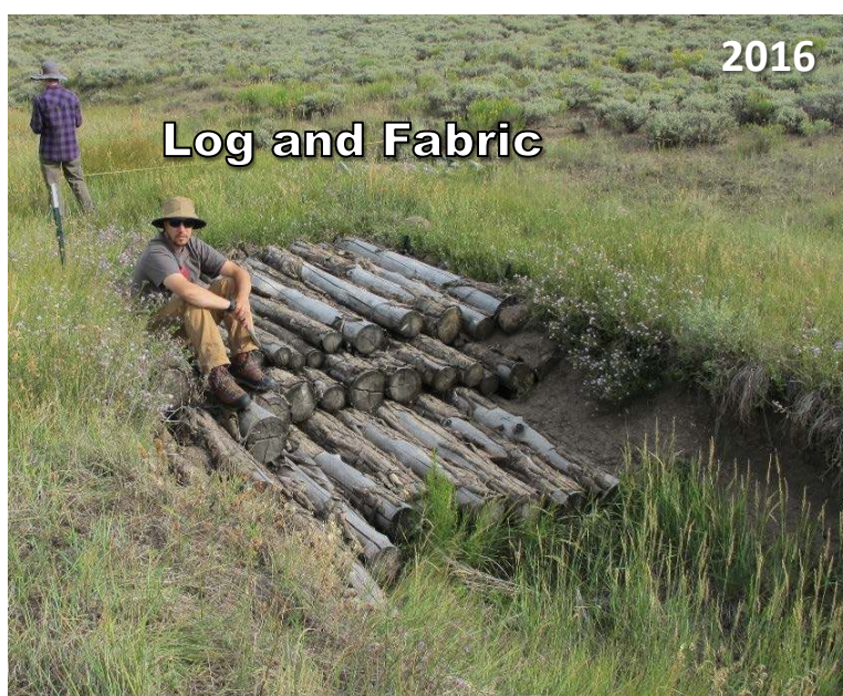
Figure 13. Log and fabric structure for treating headcuts before (top) and after (bottom) installation. Photos by: Renee Rondeau
