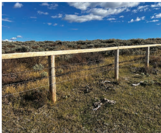
Pole top fence. Sublette County, Wyoming.
